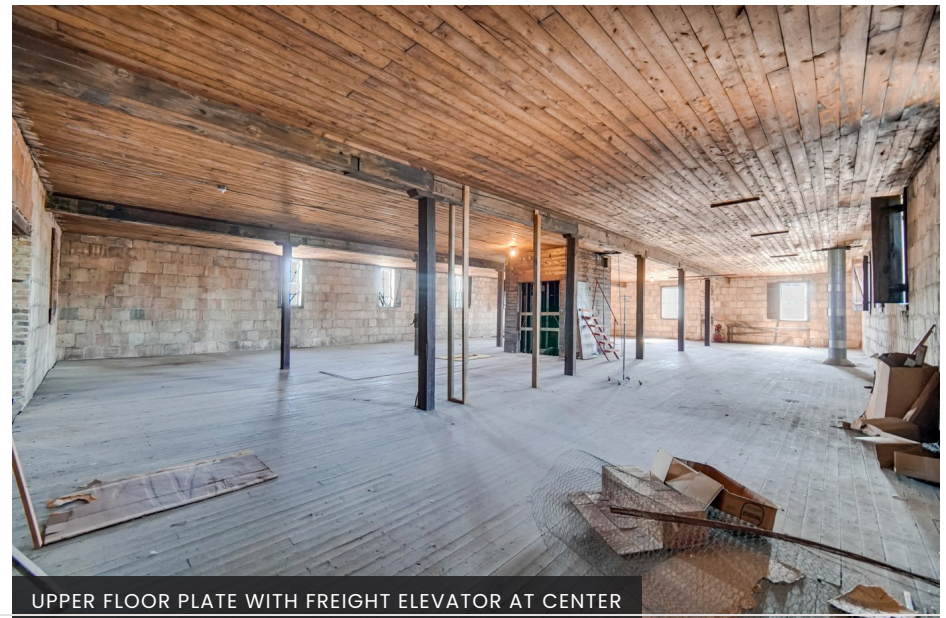
HEAVY-TIMBER STRUCTURE AND WOOD CEILING
