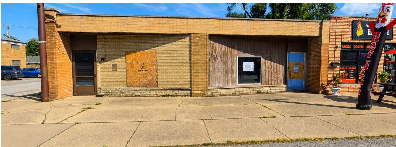
EXTERIOR ALONG 147TH STREET, SHOWING STOREFRONT TO BE RESTORED
